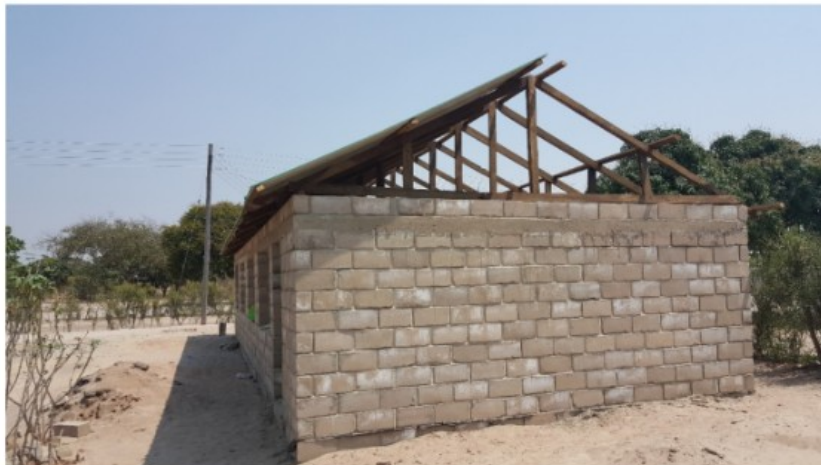
Village chicken house in Mongu being roofed (Second project phase) ( 10 x 6 Meters)
