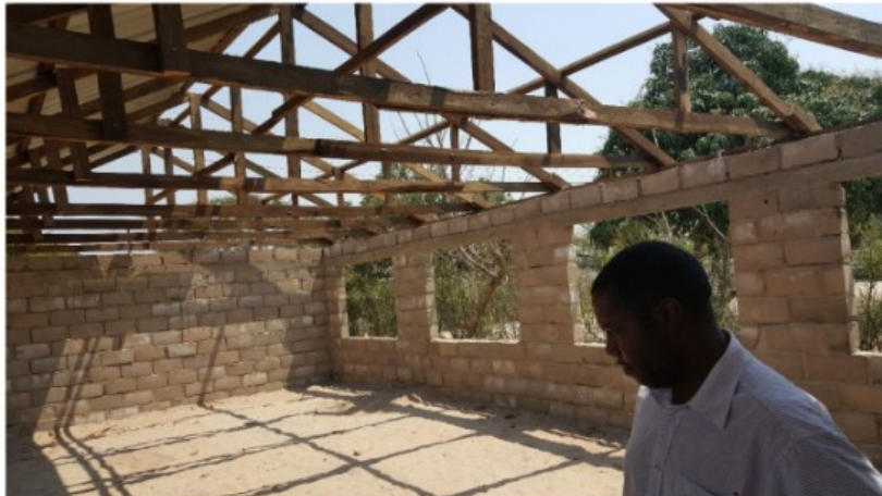
Village chicken house under construction in Mongu (Second project phase)
